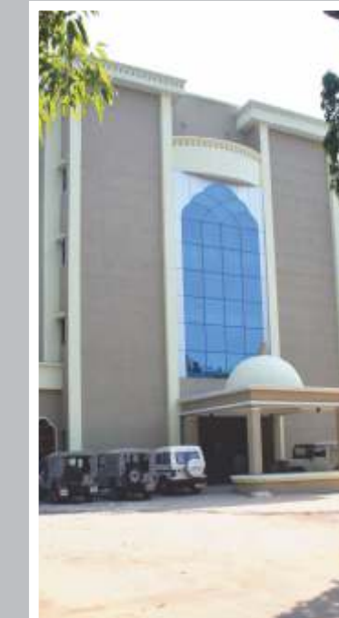
Atomic Minerals Division - Office Complex Begumpet, Hyderabad
